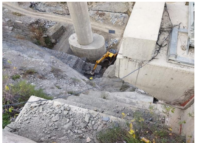
Figure 10: Pier Protection Work at Bridge -138
