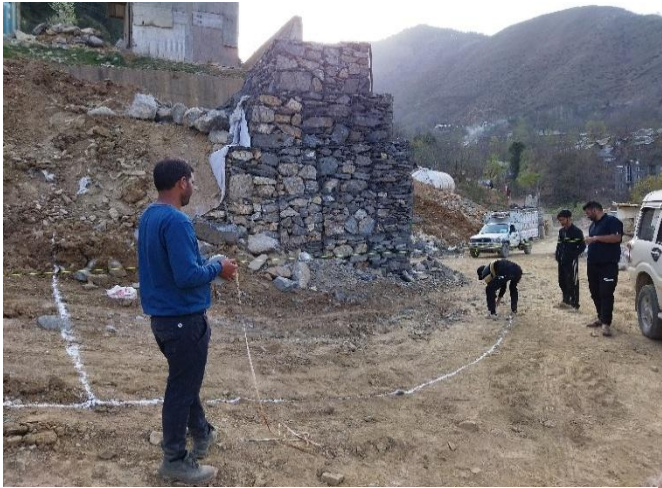
Figure 5: Marking at T78-P2
