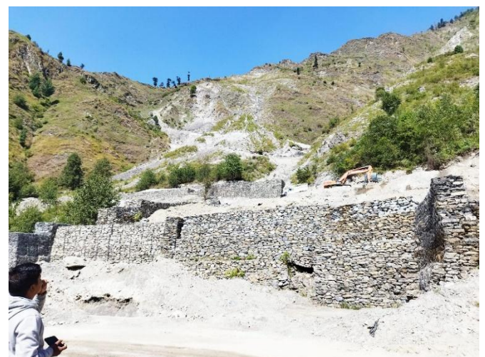
Figure 4: Erection of Gabion walls at T74R-P1
