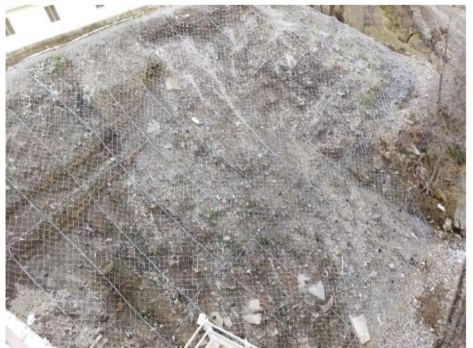
Figure 9: HEA Panel Installed at T74R-P2
