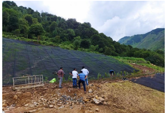
Figure 2: Inspection of Hydroseeding at T78-P2
