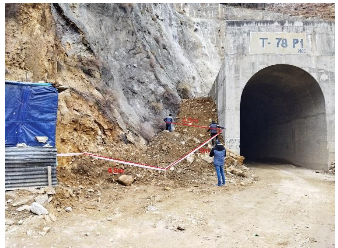
Figure 3: Marking at T78-P1
